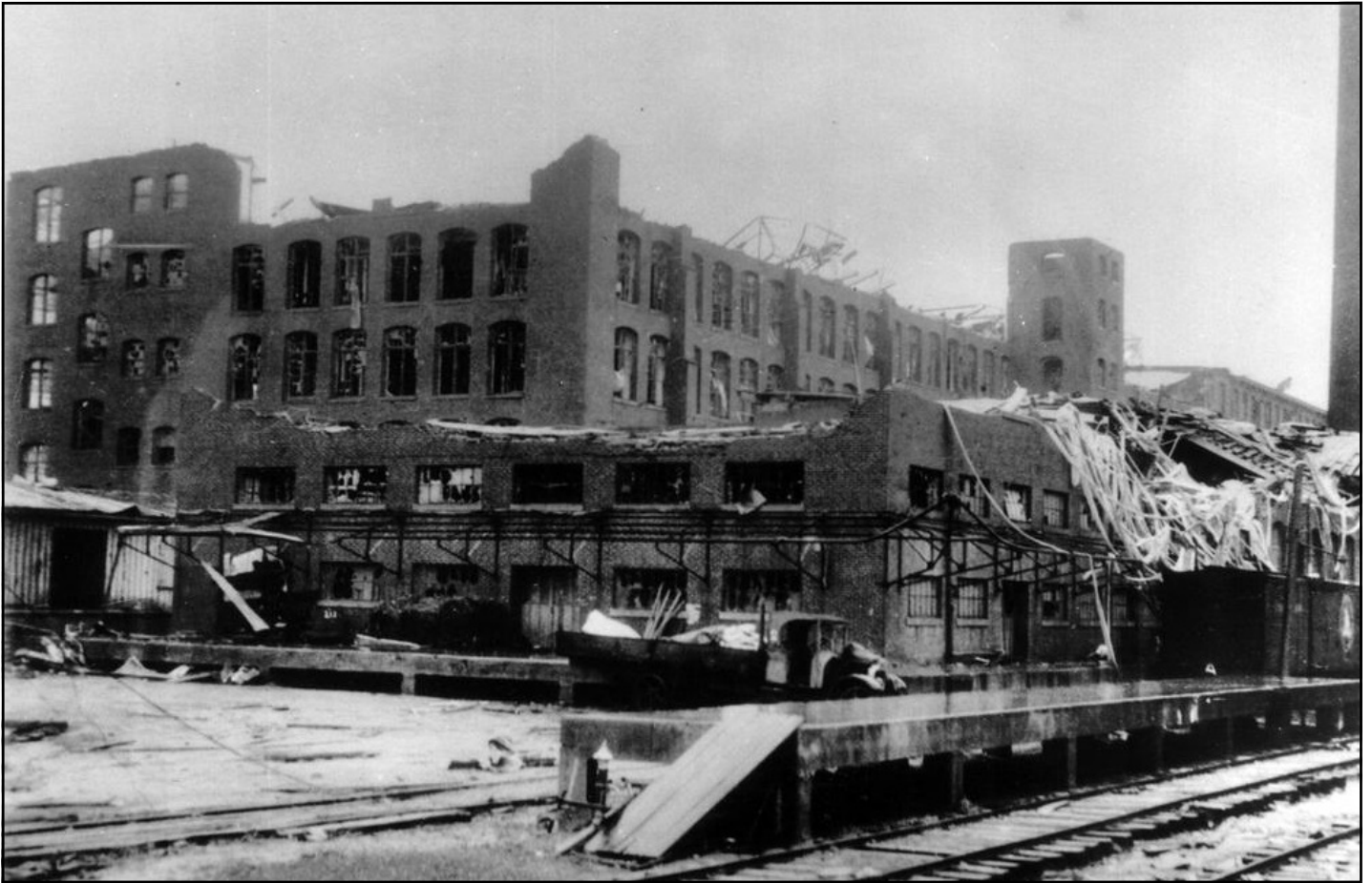
Contemporary 1936 Newspaper Photo of Damage to Pacolet Mills No. 6
